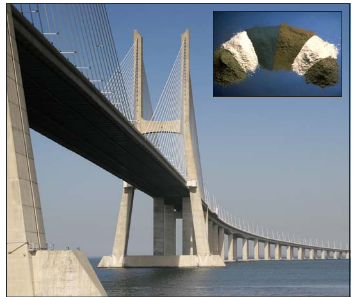
Figure 6. Recycled industrial byproducts such as fly ash, slag and silica fume (inset) are used to enhance durability of concrete by decreasing permeability and cracking.
